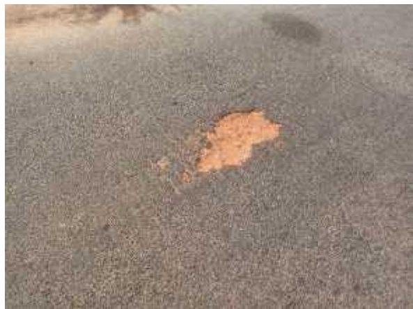
Fissures (nid despoules)
